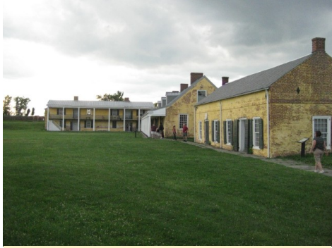
Buildings at Fort Mifflin
